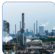
Large Plant Area
